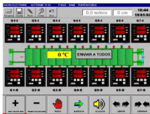
Temperature control screen
